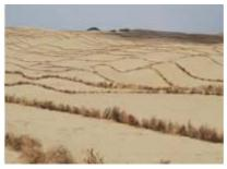
A typical model of horizontal pattern of wind break put over a very active sand dune area in Jaisalmer district
