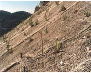
Jute netting is used to protect the bare land slope from the direct impact of rain thereby reducing splash erosion. It retains soil moisture, increases infiltration rate, enables vegetation to establish, and reduces landslides along roads.
