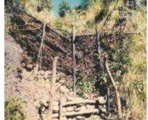
Figure 6.8: Brushwood check dam with rope tied post, wire mesh tied to post, and wooden log tied posts
