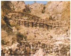
Figure 6.12: Live crib wall for riverbank and stabilization of steep slopes
