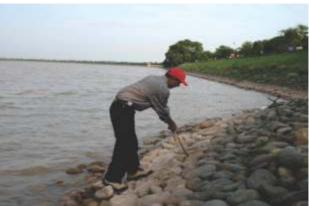
Figure 6.11: Rock revetment for shore protection of a large water body
