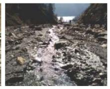
Figure 6.9: Debris deposited by FCCD and centralized flow in stream after a flash flood
