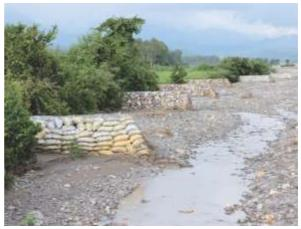
Figure 6.16: River bank protection by bio-engineering measures of gabion spurs and vegetation
