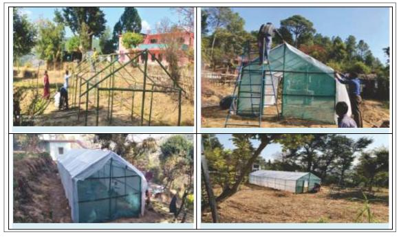
Figure 10.2: Construction of low-cost bamboo polyhouses in the village cluster
