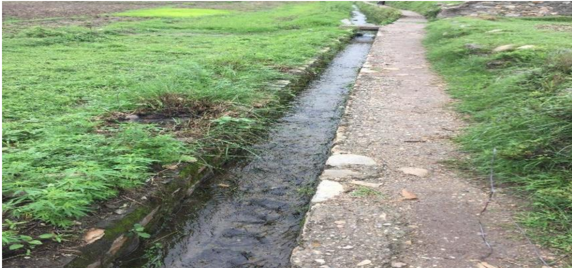
Figure 4. Traditional Gul channel irrigating terraced agricultural fields in Kumaon
