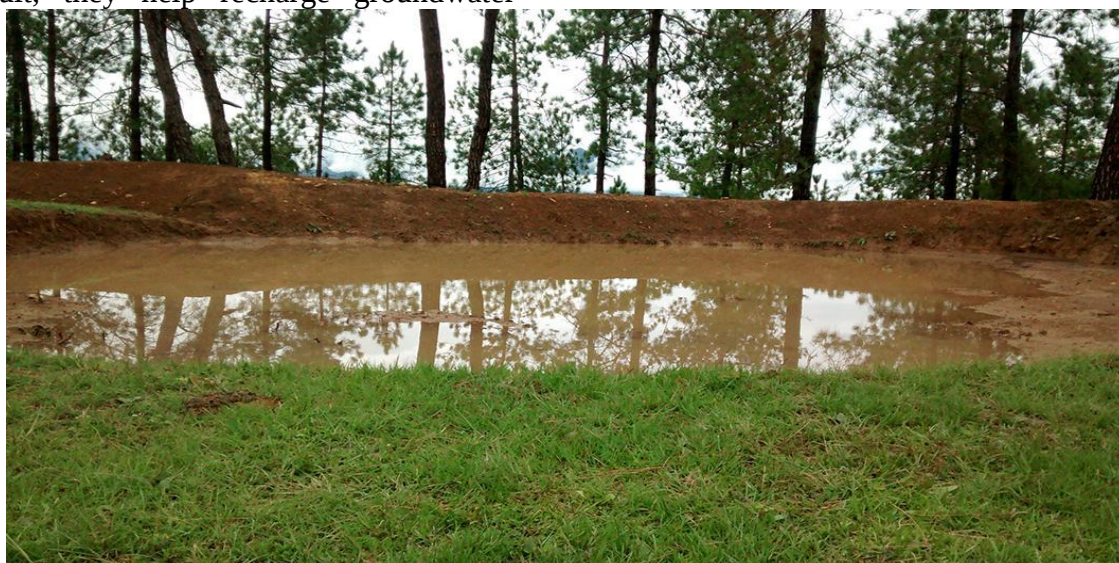
Figure 3. Chal/Khal system used for rainwater harvesting and groundwater recharge.
