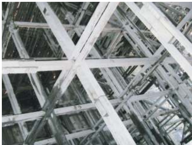
Timber structure inside the cooling tower
