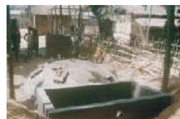
Installations of gobar gas plant
