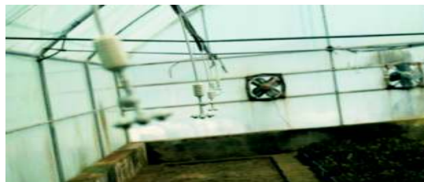
Fitting & Fixing of Micro-fogger in Hi-Tech Nursery at R&D Centre, Rajkot (Gujarat)
